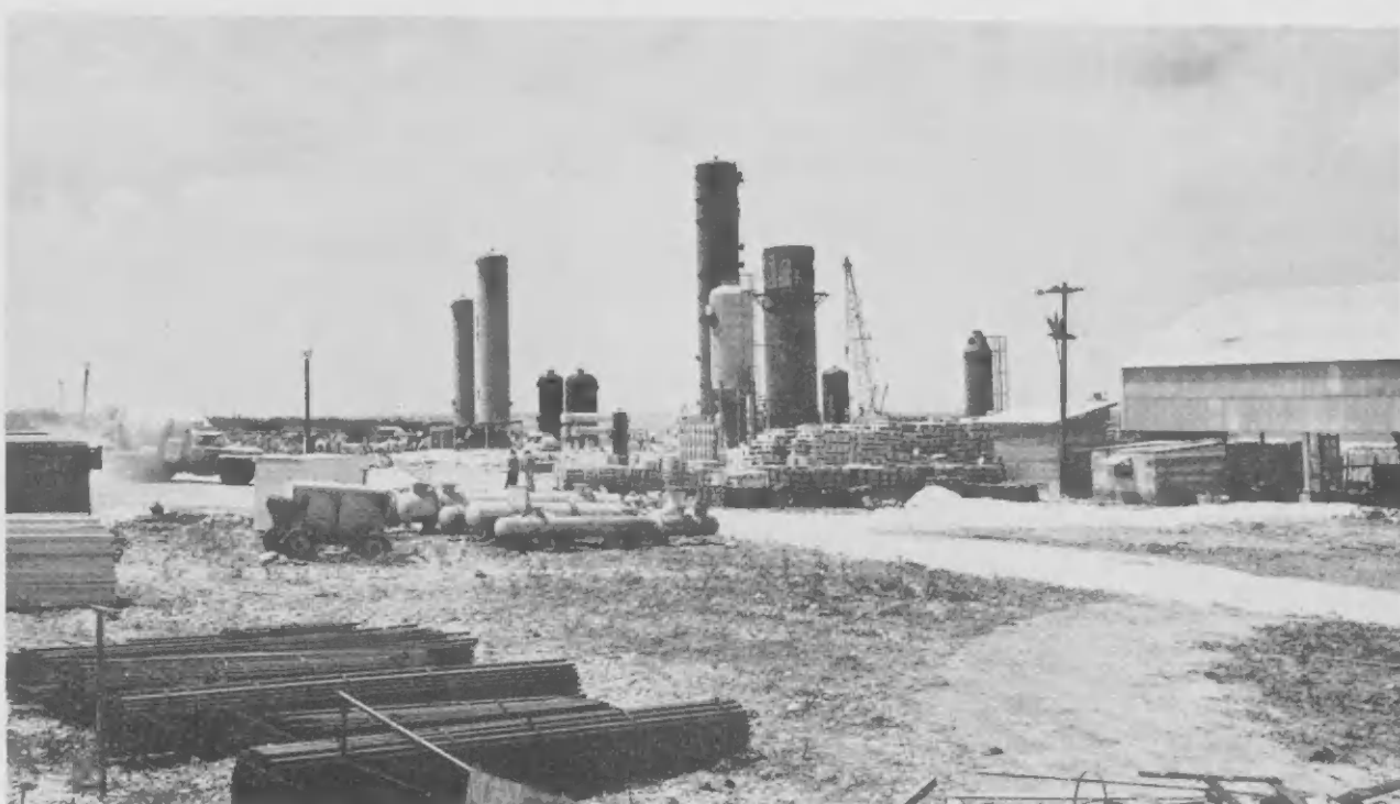
AT THE Barcadera industrial site, a heavy-duty crane positions a first-stage absorption tower. The big tower is one of many process units that will make up the Antilles Chemical Company plant. It weighs nearly forty-three tons and stands nearly sixty feet in the air.
